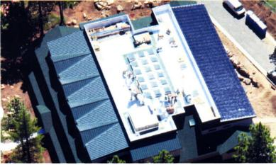
The 31.5-kilowatt photovoltaic system has 900 PV roof tiles and nine 3,500-watt inverters with combiner boxes.
