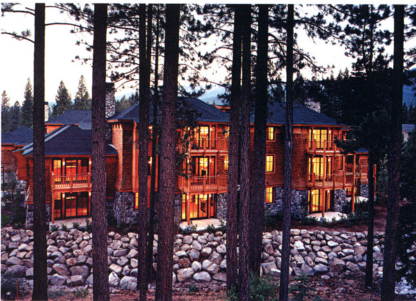
Photo courtesy of Krump Construction, Inc.
