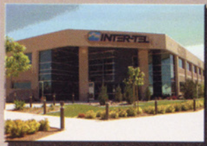
Intel Operations Center
