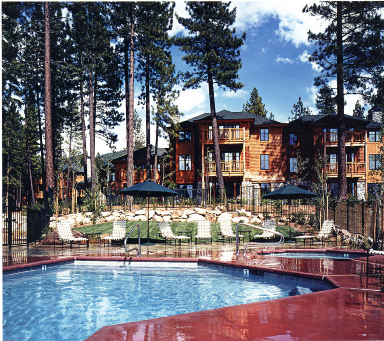
Photo courtesy of Krump Construction, Inc.
