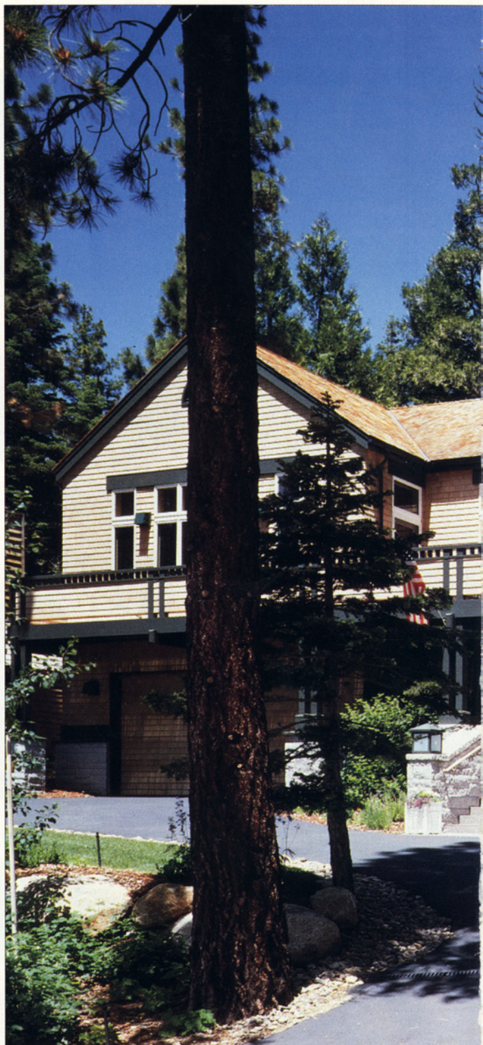
▲ This custom home derives its timeless appeal from natural materials skillfully applied, including granite front steps, red cedar shingle siding with a light stain, and, in a concession to harsh weather, vinyl-clad wood windows.
