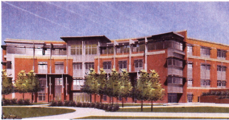
The exterior skin is a complex combination of brick, metal panels and glass because each façade is different depending on its orientation to the sun. Photo courtesy Collaborative Design Studio.
